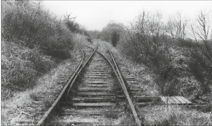
The lead into Carter's Siding (left) from the erstwhile Wimborne loop, looking south west, 24th April 1965. A former ground frame had been replaced in the 1930s by the single point lever (right foreground). The headshunt continued for about four chains behind the camera. Nature is quickly reclaiming its own. Colin Caddy
