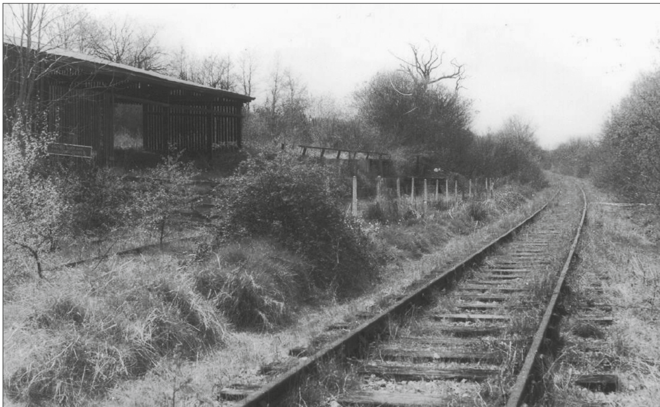
Carter's Siding (left), looking south west along the remains of the S&D's Wimborne loop towards Corfe Mullen Junction, 24th April 1965. Note the transshipment shed, loading dock and entrance gate with notice saying: 'ENGINES MUST NOT PASS THIS BOARD'. Colin Caddy
