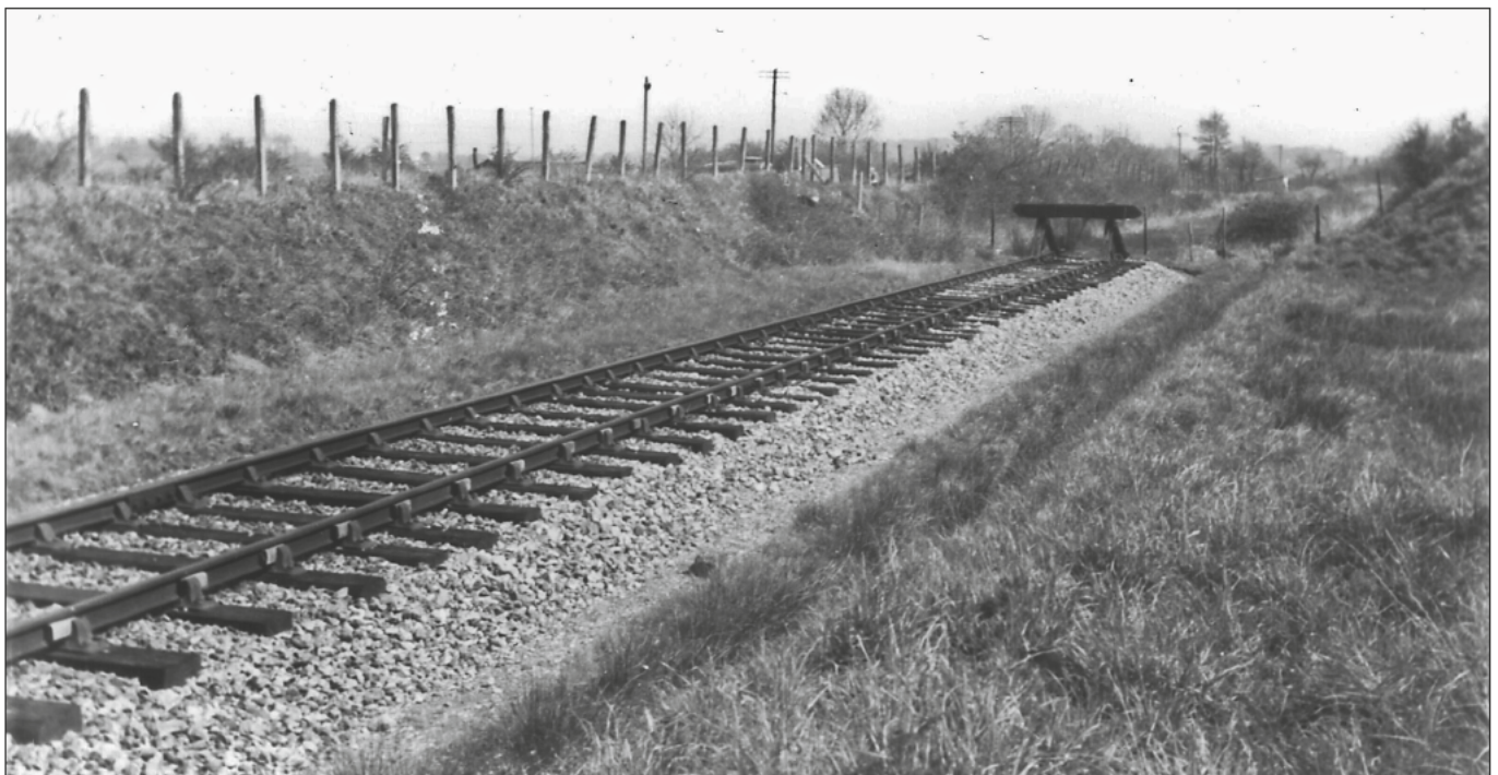
The stub end of the erstwhile Wimborne loop, looking north on 17th April 1949. This formed the headshunt for working Carter's Siding. The loop had been cut back to the buffer stop (61ml 21ch from Bath Junction) in 1933. Unknown; courtesy R. K. Blencowe Collection, ref 19963.
