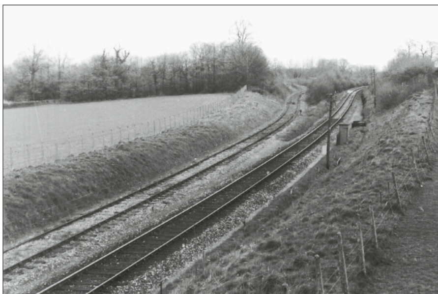
The divergence of the Wimborne line (left) and Broadstone line, looking east from Corfe Mullen Junction Bridge, 24th April 1965. The goods train serving Carter's Siding would have initially pulled up on this section of the Wimborne loop clear of the junction and ground signal, before uncoupling the portion to be shunted to the siding. Colin Caddy
