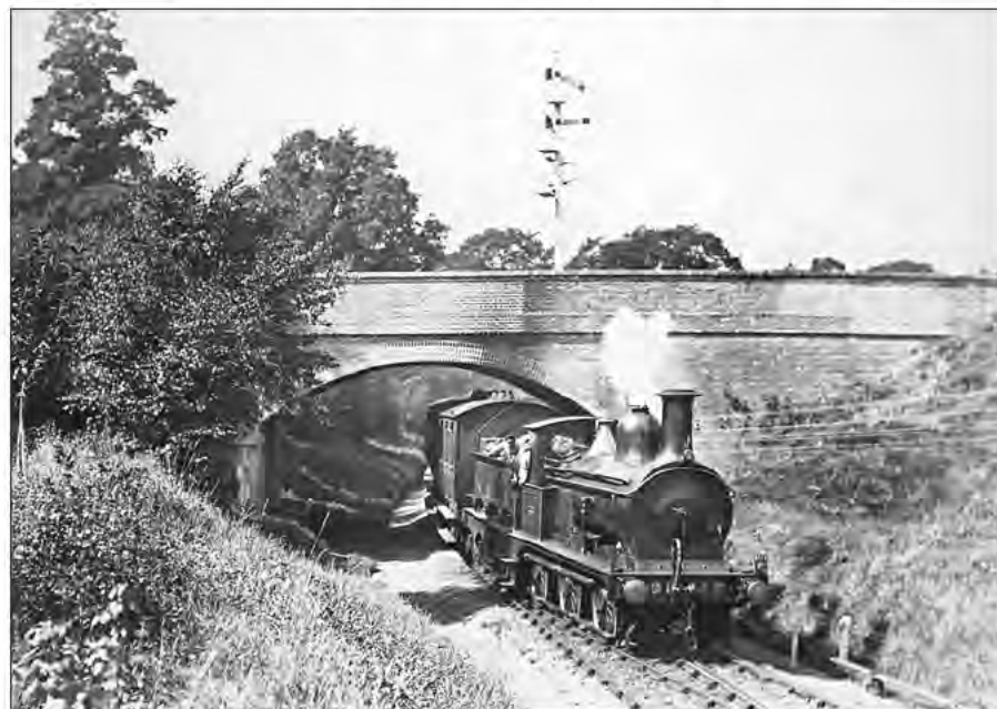
A Vulcan ('Scottie') 0-6-0 No. 56 and Wimborne-bound train pass under Oakley Road Bridge at MP 63 and over Wimborne Single Line Junction, circa 1900. Note the tall junction signal, to allow good sighting from the S&D signalbox behind the camera. The bridge carried the main Wimborne-Poole road over the S&D and was clearly built for double track. A head-on collision occurred west of the bridge in 1866. Wimborne Bypass now passes through this site to the left, under a modern concrete bridge.
