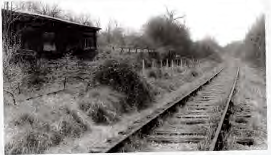
Carter’s Siding, looking SW towards Corfe Mullen Junction, 1965. Note the siding passing through the gate alongside the transhipment shed and loading dock. Birch saplings indicate the lack of use since 1959. The warning board (centre left) was the one the author removed in Summer 1965. Colin Caddy
