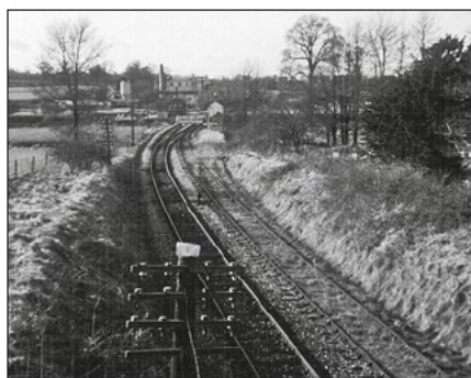
Corfe Mullen Junction, looking west from Bridge 223, May 1968. The grassy stub of the S&D's Wimborne loop to Carter's Siding awaits lifting; it was gone by Summer 1968, the Blandford-Broadstone line alongside being removed in 1969-70. Note the catch siding off the Wimborne loop, which ended in a sand drag. Peter Russell
