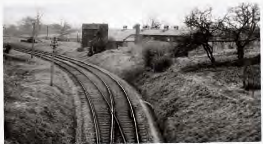
Wimborne S&D Single Line Junction looking east from Oakley Road Bridge, with the third S&D shed, water tower and LSW lines in the background. Dated 1931, the shed had been closed since 1923, yet appears in good working condition. The S&D signalbox, closed 1928, has gone, its site marked by bushes near the water tower. The S&D Up line looks well used. The orchard (right) was at the bottom of the S&D hostel gardens.
