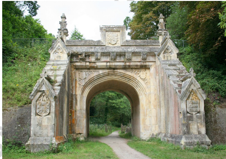
Fig. 1 Bridge 77 (2010). Photo: C. Divall.
