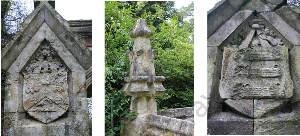
Fig. 2 Details of Bridge 77 (2016-18). Photos: C. Divall.
