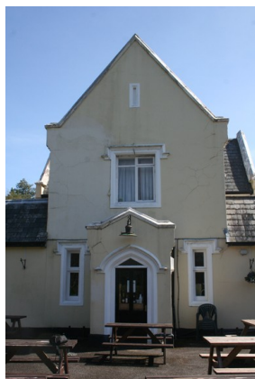
Seen here in 2015, the entrance porch with the booking hall beyond survives at Holmsley, although the oriel window has gone. Render obscures the original brickwork. Photo: C. Dival.
