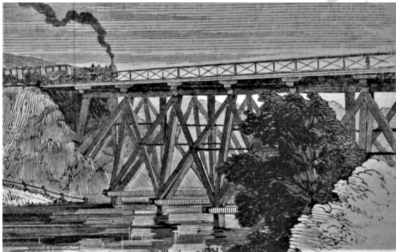
Fig. 1. The Stour viaduct. Extracted from Illustrated London News (5 June 1847).
