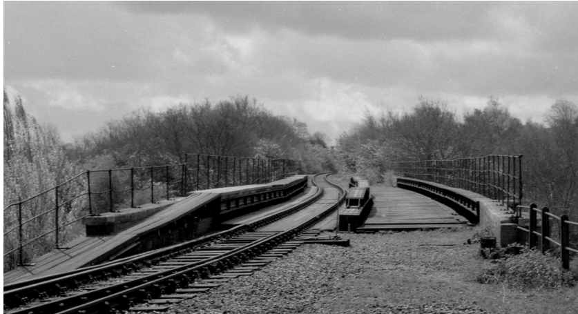
Plate 3. The girder reinforcements, April 1977. Photo: C. Divall.
