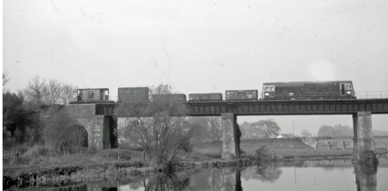
Plate 5. Bridge 76, 10 April 1974. Photo: C. Divall.
