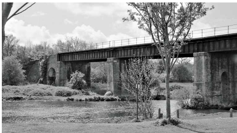
Plate 1. Bridge 76, looking SW towards Poole, April 1977. Photo: C. Divall.
