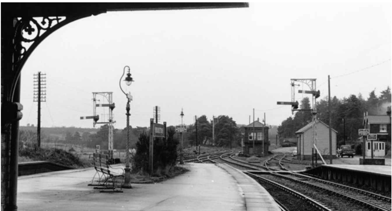
A 1965 view of Broadstone station, looking north from the island platform, showing the 'crossroads' nature of the junction. The S&D line curves its way through the straight line formation of the Ringwood-Hamworthy Junction route. [Photo by Peter Barnfield/S&DRT collection, ref. WSHSD_2015_50_14.]
