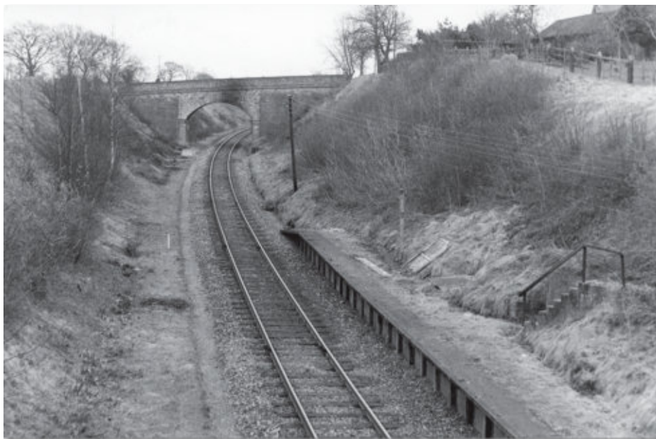
In this eastward view from the early 1960s, the double-track formation is once again clearly evident, including the double-width arch of Lamb's Green Bridge in the background. After the halt closed in 1956, the curvature of the single line was eased slightly away from the platform edge, possibly when the flat-bottom rail was laid.
