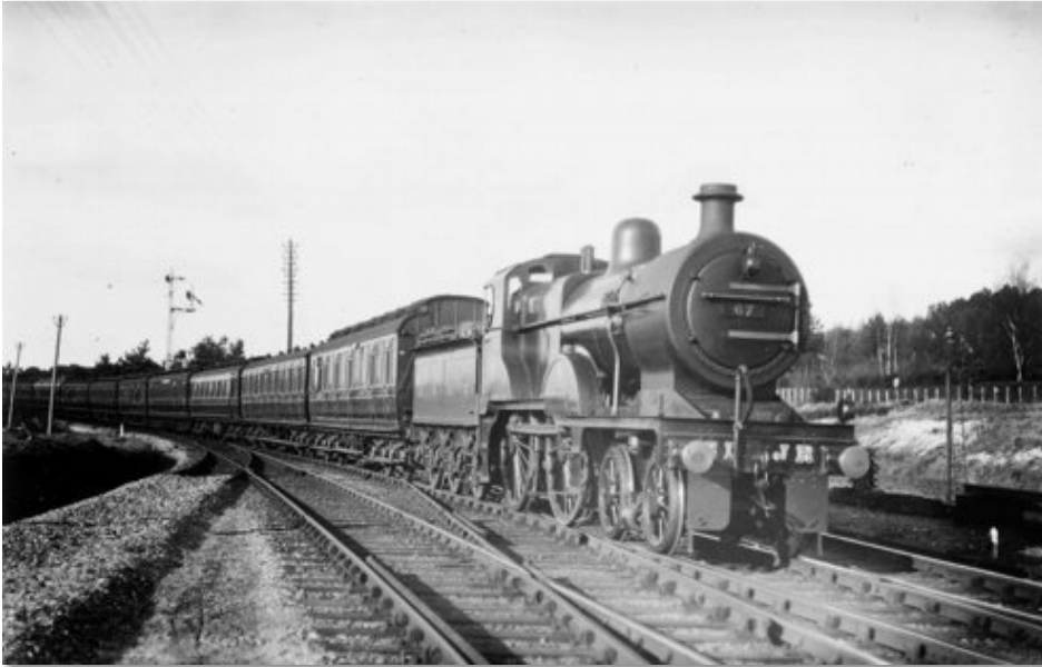
Here we see the double track at the junction merging into the single line of the cut-off just north of the junction in the early 1920s. The second (Up) line would have been added beyond the coaches. Note the gravel (ballast?) trap to the left. This alignment had earlier held a siding extending 500 feet towards the north end of the Up (Hamworthy) platform, and possibly used for berthing 'tail-end' traffic off Up trains, pending moving to the yard. S&DJR blue-livery 'large' 4-4-0 No. 67 (later LMS No. 324 and BR No. 40324) brings a Bournemouth-bound train into the station. [Photographer unknown; R. J. Essery Collection, via S&DRT.]
