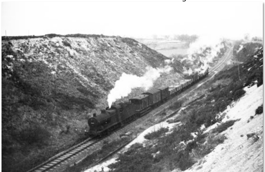
A spectacular and rare westward view from the top of the cutting's north-east side, this shows the vast extent of the earthworks needed for the single-line cut-off and its proposed doubling (a stark contrast to the gentle Stour Valley route of the original Wimborne line). This could be an industrial landscape except for the light tone of the exposed heathland minerals – simply sand and gravel. Landslips were as frequent here as at Ashington Cutting, hence the wide cutting, but no serious revetment was provided beyond the partial low fencing visible on the Down side. The track alignment can be seen running back to the summit near Ashington Bridge. Class 4F 0-6-0 No. 44560 is coasting down-grade at 11.15 am with the 6.35 am Evercreech Junction-Poole goods. 6 April 1964.
