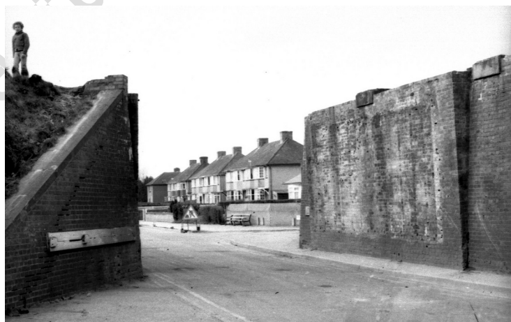
Plate 1. Abutments to Bridge 75, probably in February 1977, looking west and showing the vertical brickwork strengthening the original cast-iron spans and the bedstones for the replacement wrought-iron girders.
